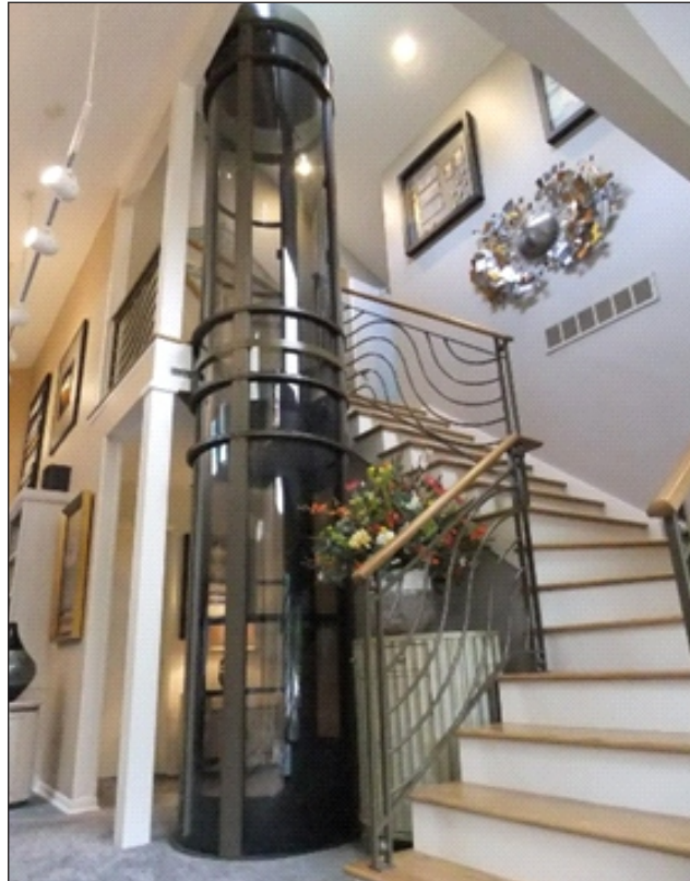
Fig. 3.1.11 Vacuum (Air Driven) home elevator
